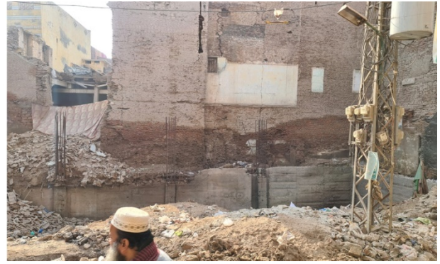
Figure 10: Left - An under-construction commercial structure adjacent to a partially demolished Early 20 th century residential building. Right - Under construction basement of a commercial structure that has damaged back walls and foundations of a Mid 19 th Century residential building. Source: Author, 2021
