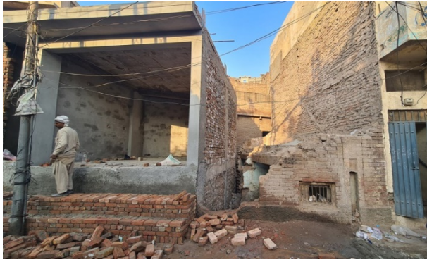
Figure 10: Left - An under-construction commercial structure adjacent to a partially demolished Early 20 th century residential building. Right - Under construction basement of a commercial structure that has damaged back walls and foundations of a Mid 19 th Century residential building. Source: Author, 2021
