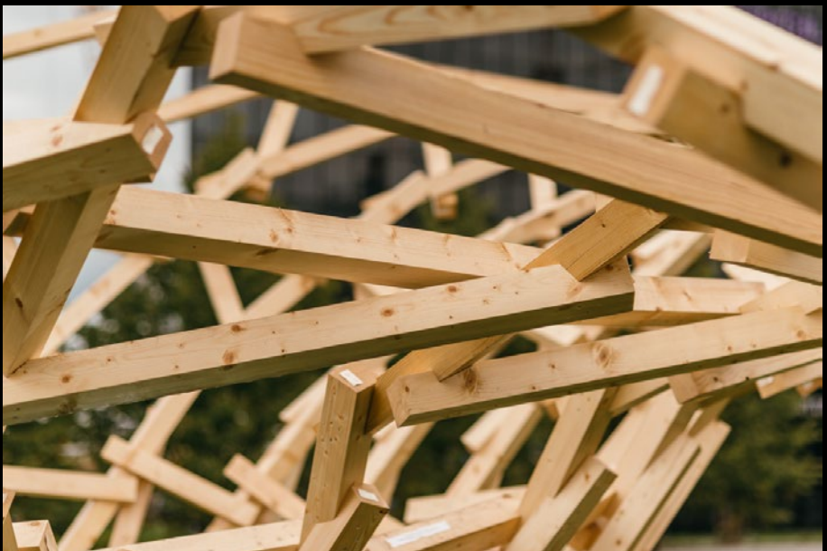
Fig. 29. Body Building installation 2015 close up – “homogeneity at a distance and near formal incoherence in detail” (Lynn 2004: 11) – the machined elements fit perfectly at seemingly random angles.
