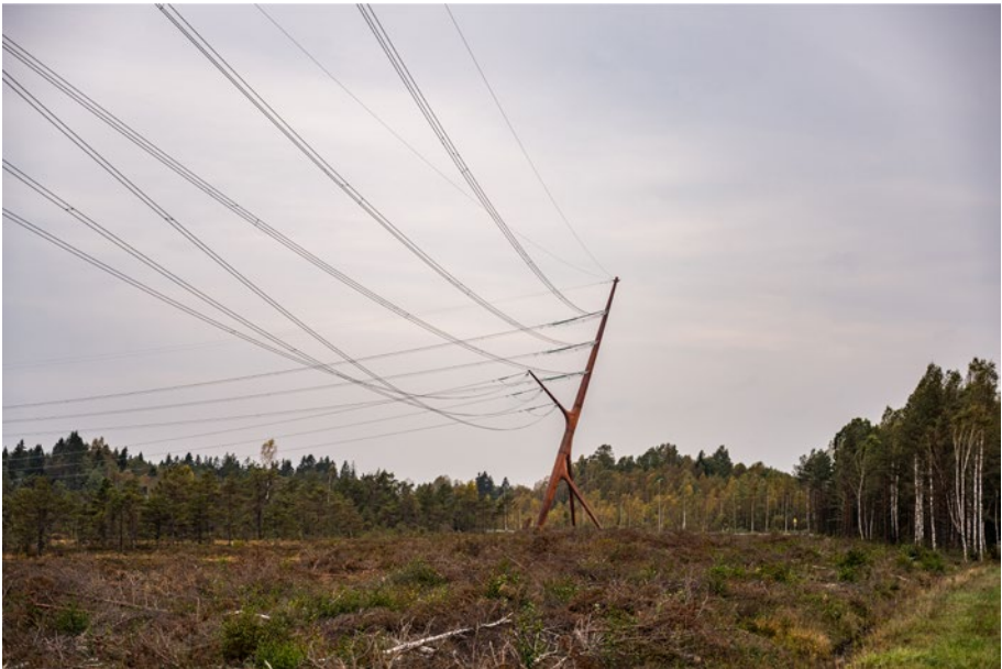
Fig. 25. Bog Fox 2016–2020, high voltage power line design pylon. Using Karamba3D, in collaboration with Bollinger+Grohmann, we set up structural and geometric checks to be able to run a genetic algorithm for material weight minimisation. Manual adjustments were made afterwards to balance additional weight versus aesthetic preferences.
