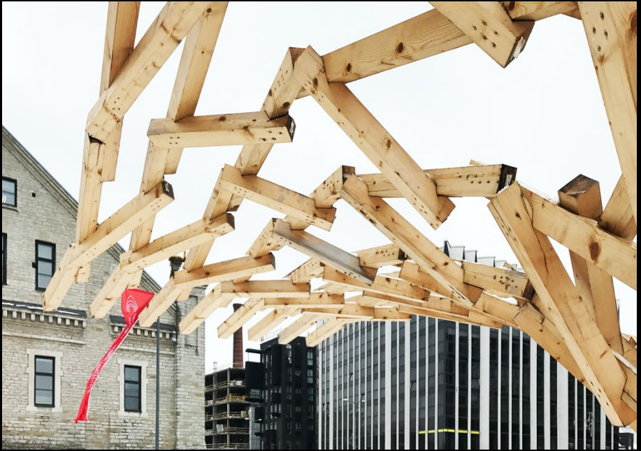
Fig. 17. Body Building installation 2015. All the pieces are unique, robotically machined with three types of algorithmically generated half lap joints.
