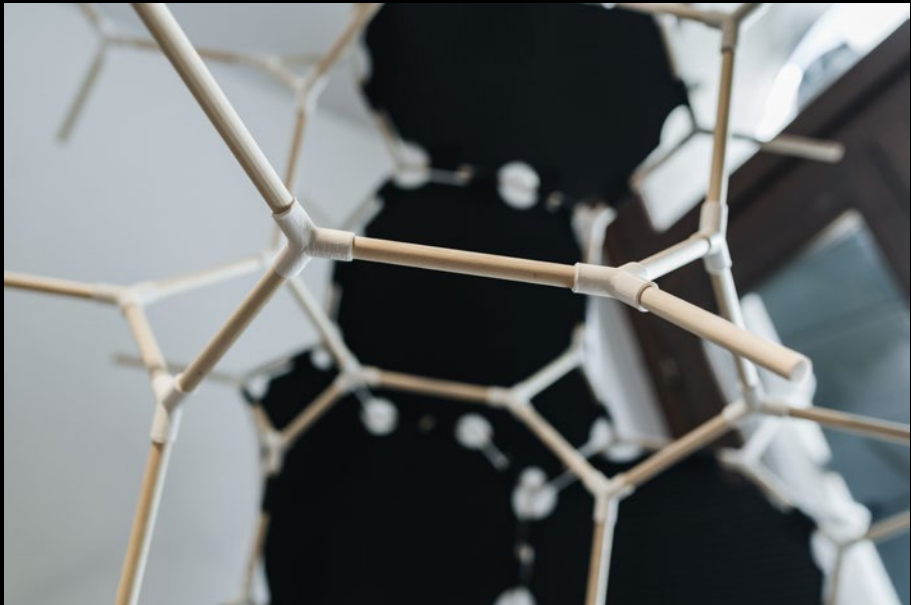
Fig. 52. PART.icular 2018, 3D printed details allow for free rotation, yet the structure finds its equilibrium in the Digital Thicket geometry.
